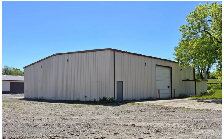
BLDG 1: 4 Motorized Overhead Doors Offering Drive-Thru Capacity
