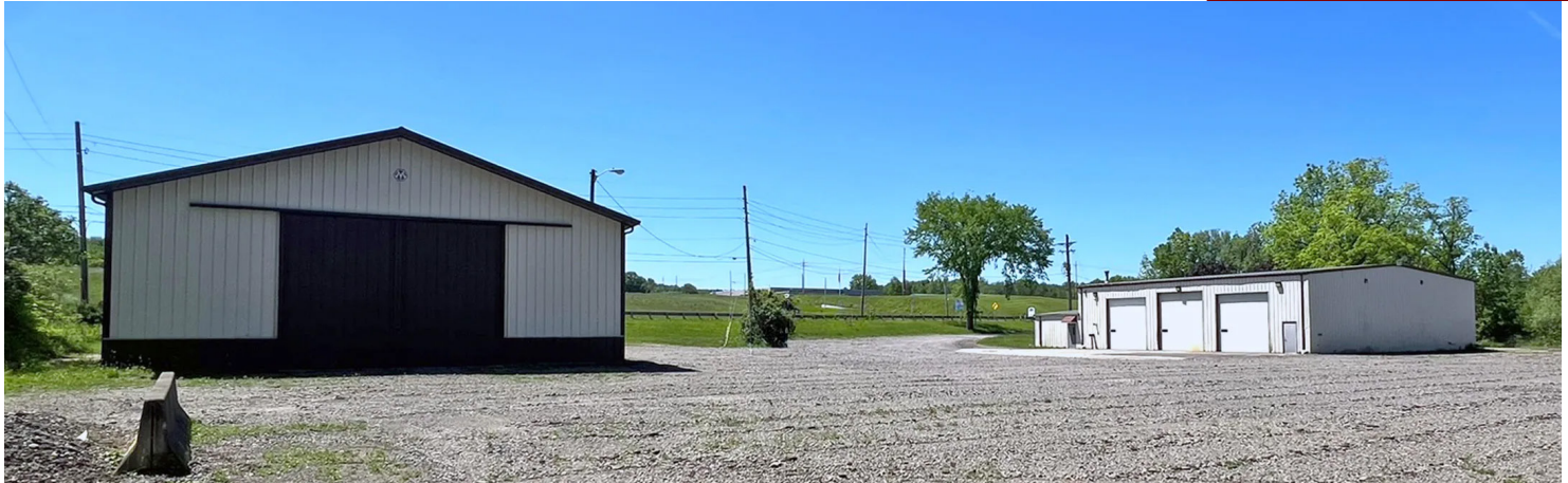
LEFT: Building 2 - 4,320± SF Unheated Pole Building Built In 1994
