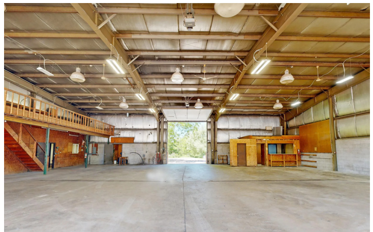
BLDG 1: Additional 630± SF Mezzanine For Storage
