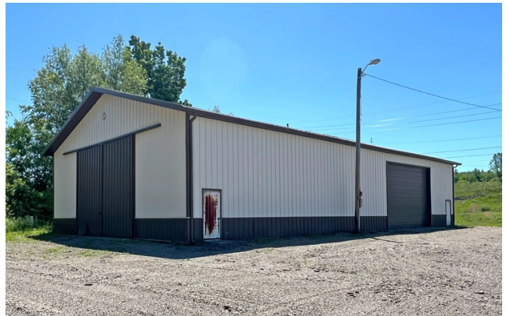
BLDG 2: 4,320± SF Unheated Morton Pole Building Built In 1994
