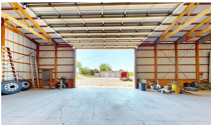
BLDG 2: 22'W x 14'6"H Motorized Overhead Door & 15'8" Ceilings Separately Metered Electric For Buildings 1 & 2
