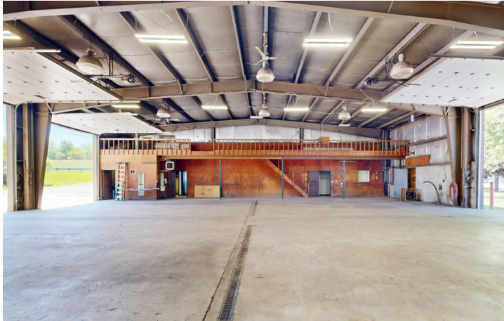
BLDG 1: 14' – 18' Ceilings, Trench Drain, Ceiling Fans & Utility Sink
