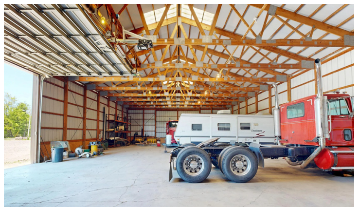
BLDG 2: 20'W x 15'H Sliding Doors At End Of Building & 100 AMP, 120/240V, Single Phase Electrical Service
