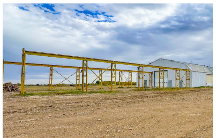
125' Exterior Crane Way
