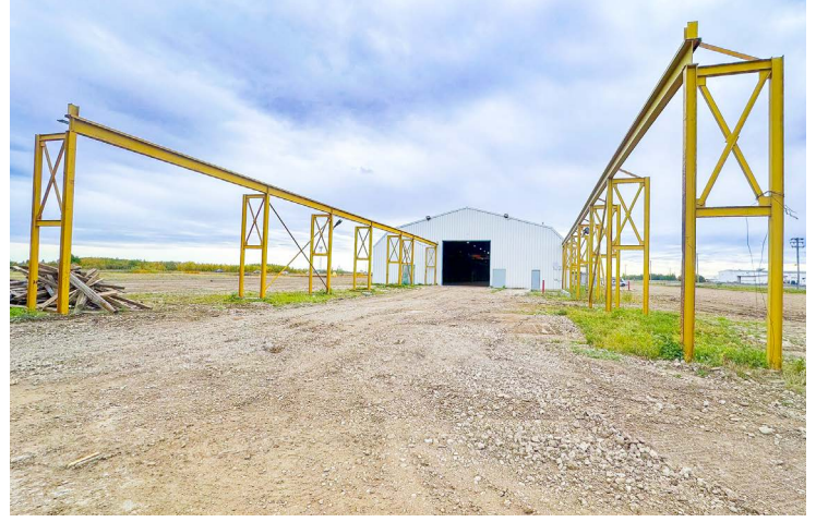
125' Exterior Crane Way
