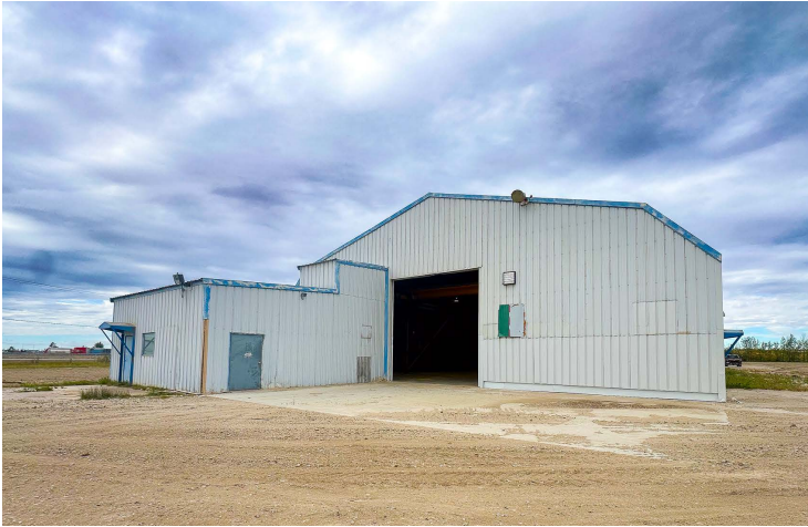
Three Point into Yard
