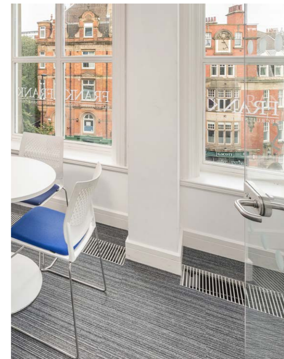
Full access carpeted raised flooring
