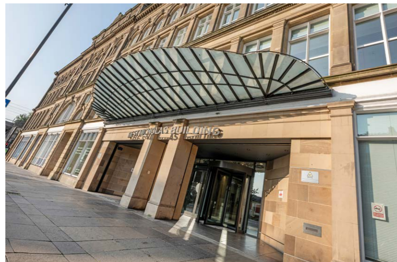
Grade II Listed Façade
