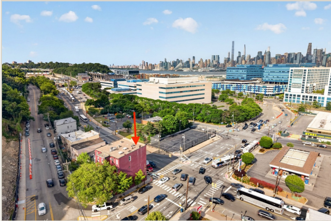
Aerial neighborhood context and property orientation.
