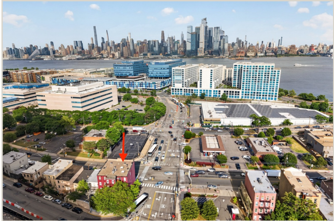
Additional aerial view toward the Manhattan skyline.
