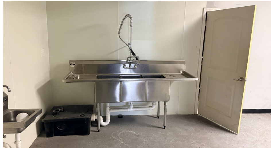
KITCHEN · 3-COMPARTMENT SINK & GREASE TRAP
