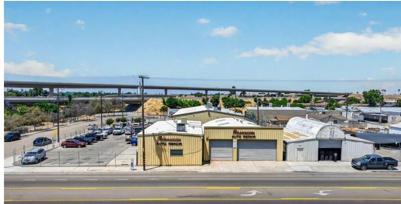
1017 N Maple Building 1
