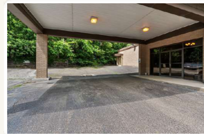
Covered exterior access
