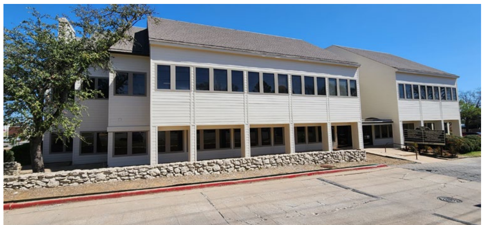
Side of Building Exterior
