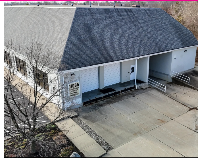
WAREHOUSE DOCK DOORS
