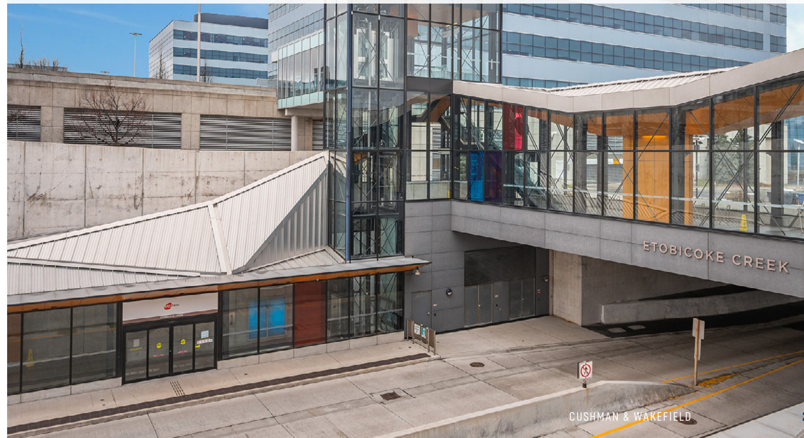
Dedicated BRT and Miway stop
