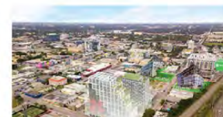
200 N MIAMI AVE Clearline 300 Units
