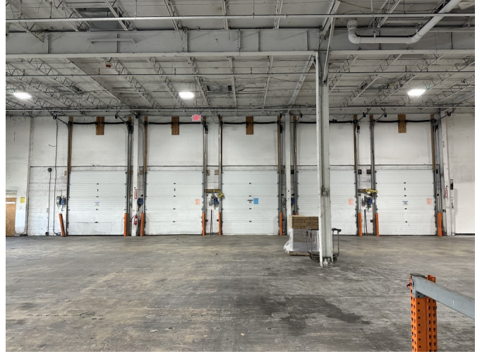
Fully Equipped Loading Docks
