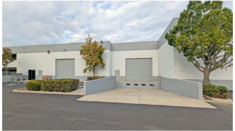
DOUBLE WIDE DOCK-HIGH LOADING
