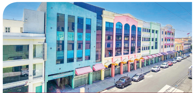
4-STORY BUILDING W/SIGNAGE
