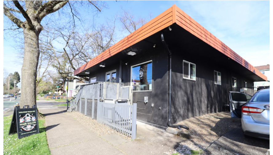
ADA ENTRY WITH LIFT ACCESS INSTALLED
