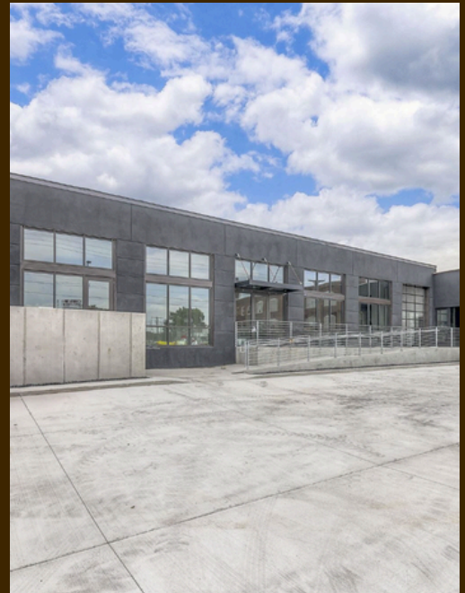
Subject Premises Photo
