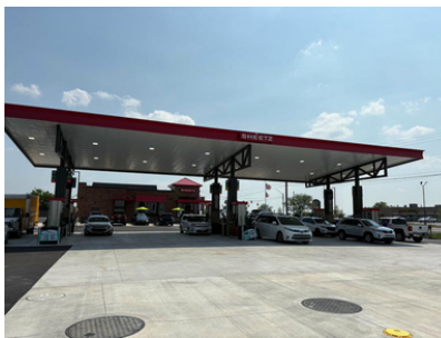
Fuel Canopy &amp; Store Exterior
