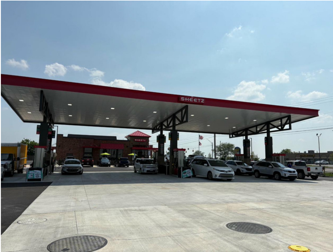
Fuel Canopy & Store Exterior
