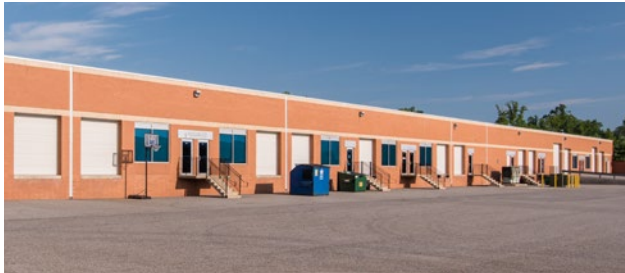
Flex/R&D dock and drive-in loading
