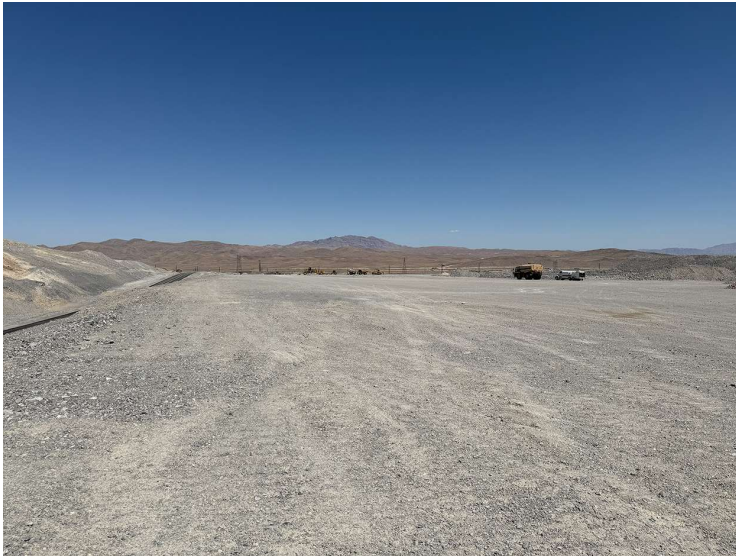
Rough graded site
