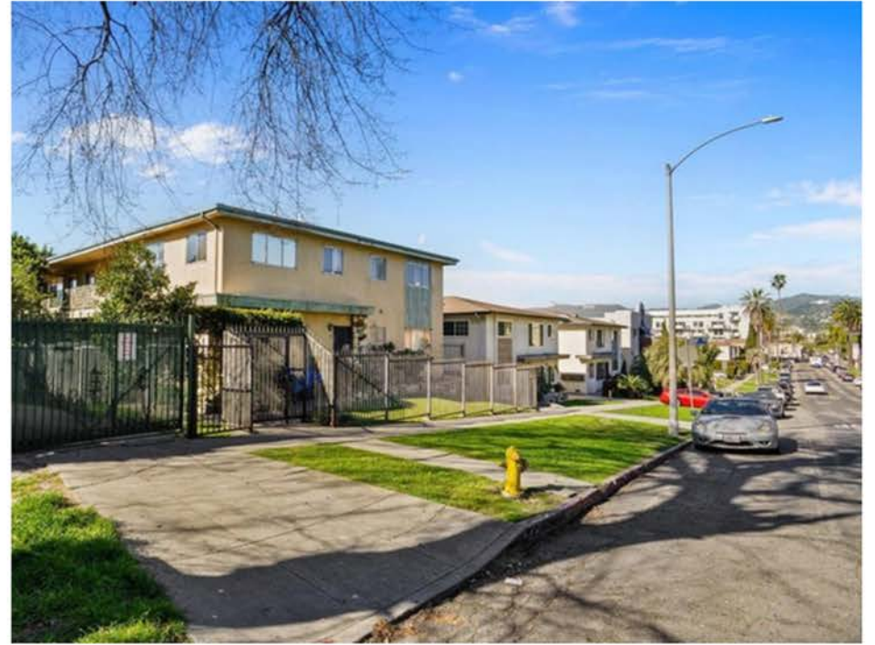
Street View of Property Facing North
