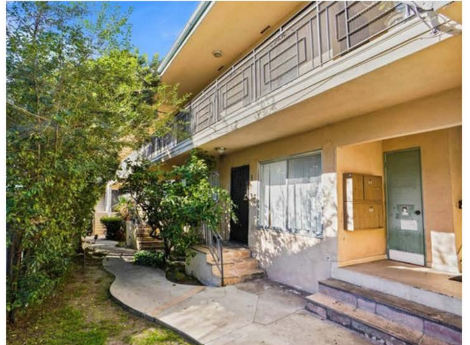
Bottom Units and Tenant Mailboxes
