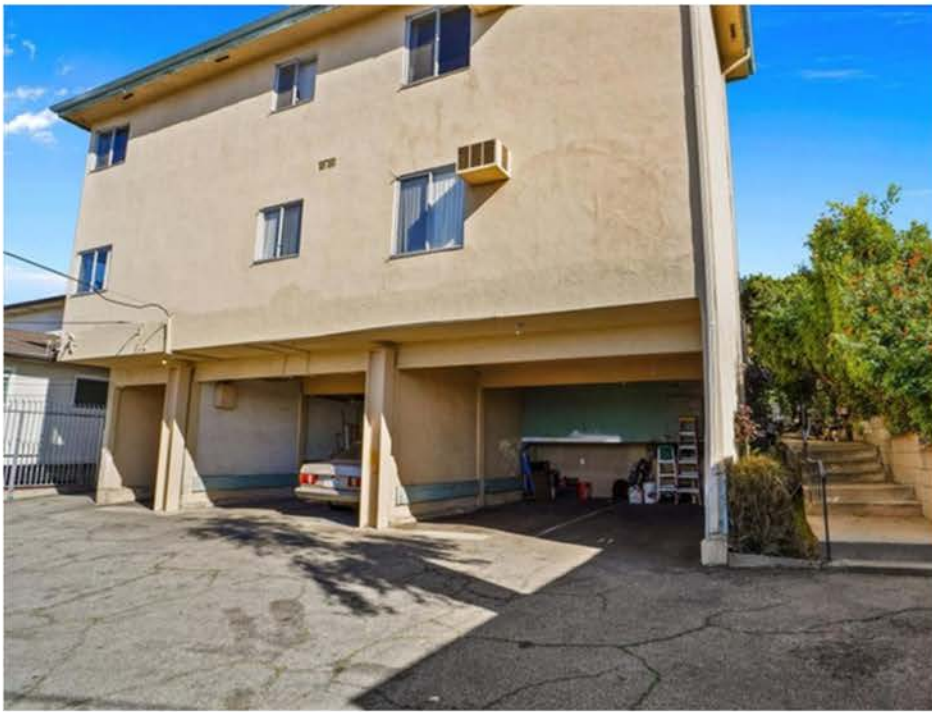
Soft Story Retrofitting & Foundation Work Done in 2018
