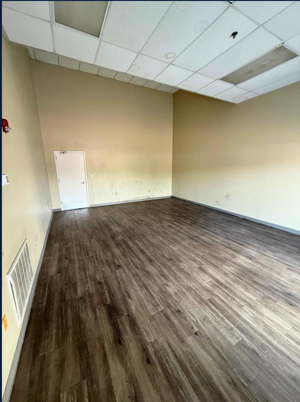
Front Office Area
