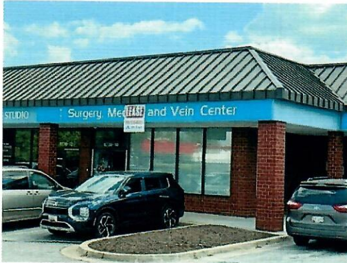
Glass storefront & Signage
