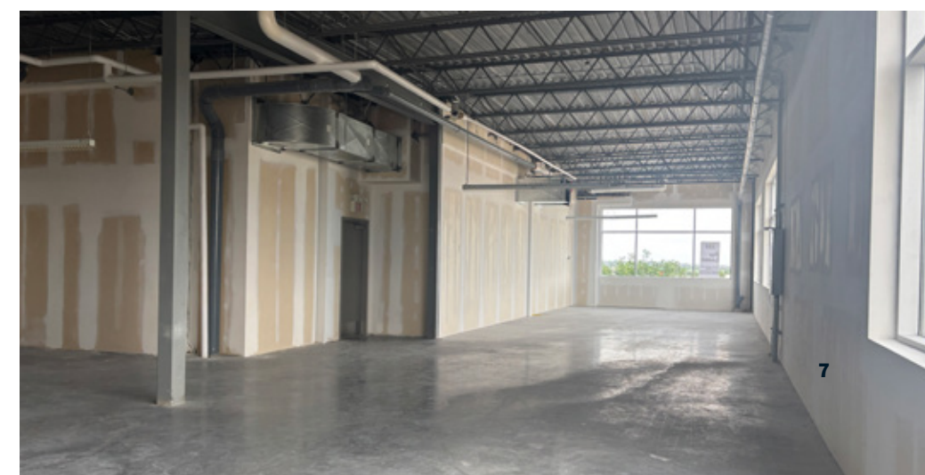
Second floor office opportunities can be combined
