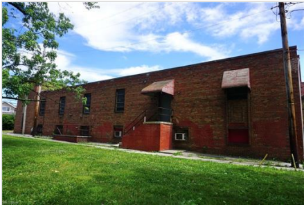
W. Side of building
