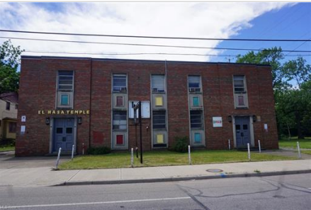
Solid brick building
