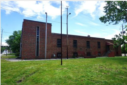
W. side of building
