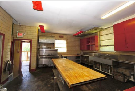
1st fl. kitchen
