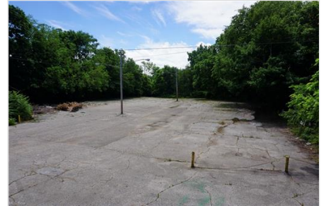
Huge rear parking lot.
