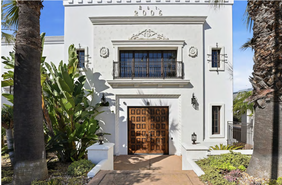
Distinctive Spanish Architectural Design & Strong Curb Appeal
