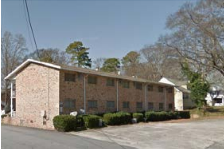
① STARFLITE APARTMENTS 3331 Sims Street, Atlanta, GA 30354
