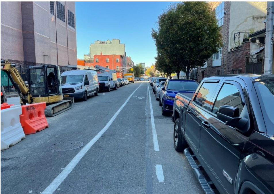
Looking west on Scholes Street
