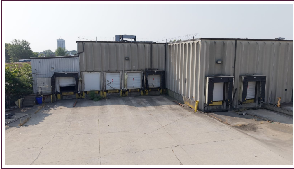
Loading dock area with multiple dock-high overhead doors
