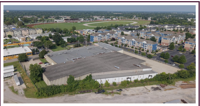
Rear aerial view along the rail corridor
