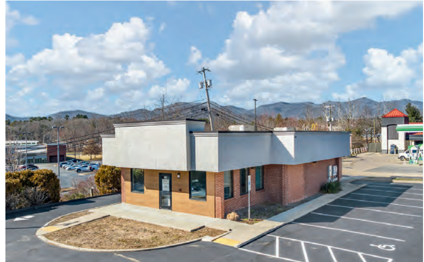
FRONT OF BUILDING
