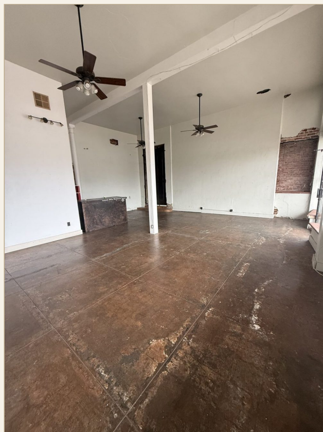
Interior — original columns and concrete, ready for a light, tenant-driven fit-out.
