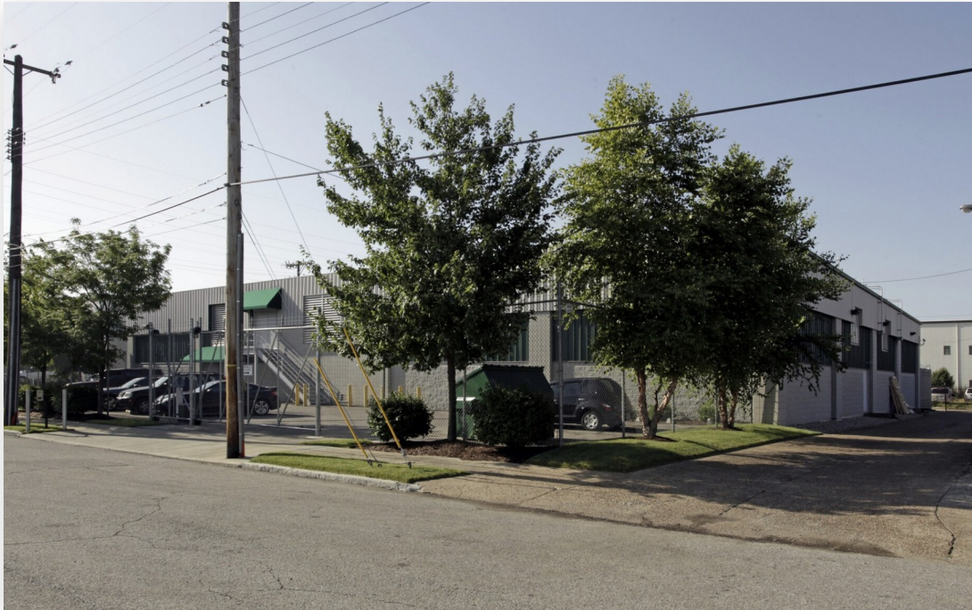
Street view: 12th Street elevation
