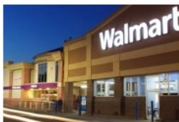
Clearmeadow Plaza 2465 Hempstead Turnpike East Meadow, NY 11554 Property Size: 208,000 S.F.
