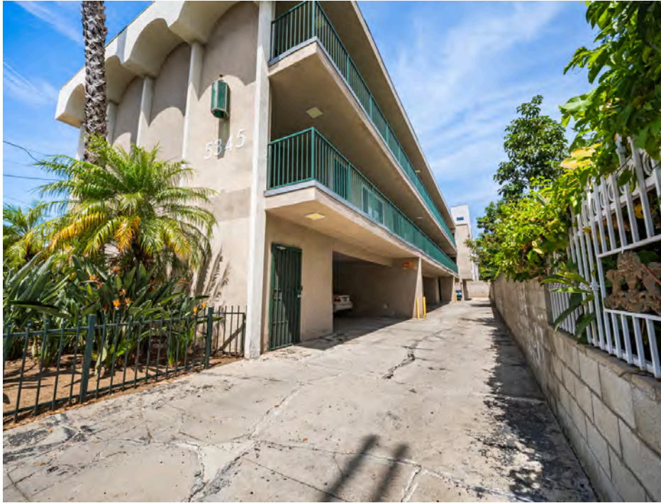
Front of Property with Carports
