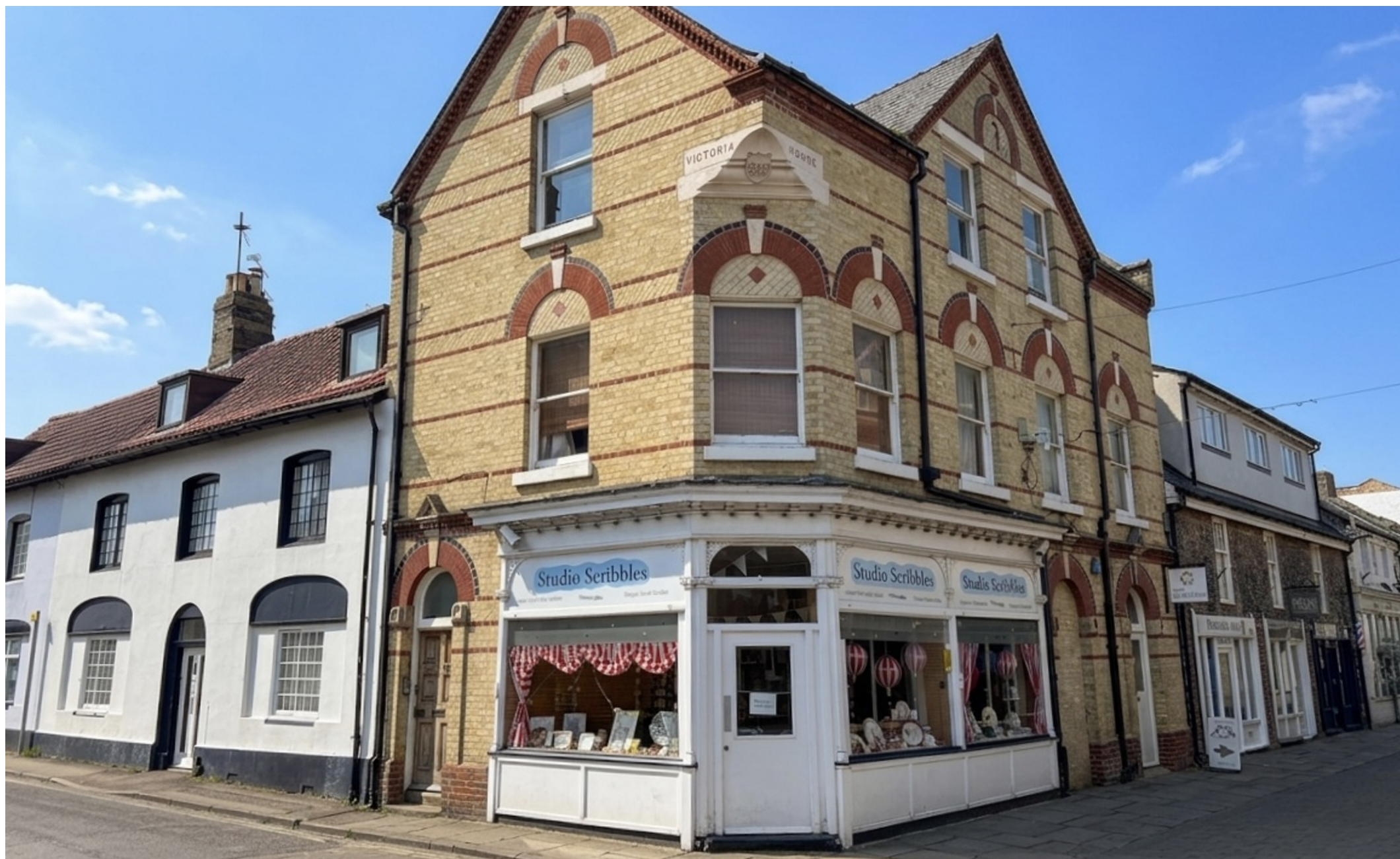
Victoria House, 2 Park Lane, Newmarket
