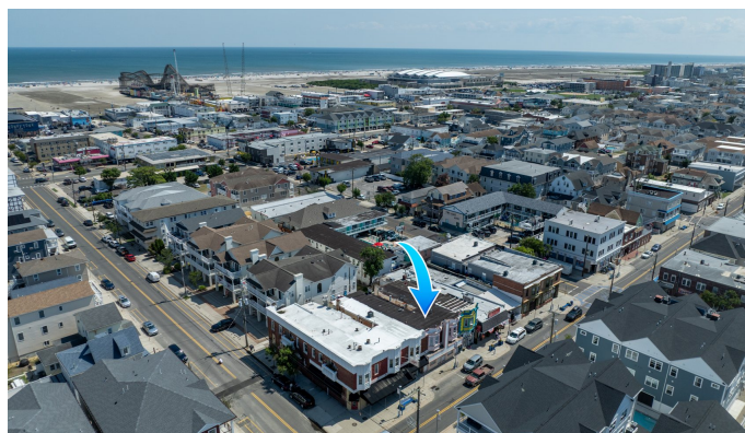
AERIAL CONTEXT — SUBJECT MARKED; BOARDWALK &amp; OCEAN BEYOND
