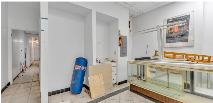
STOREFRONT INTERIOR TOWARD THE STREET
