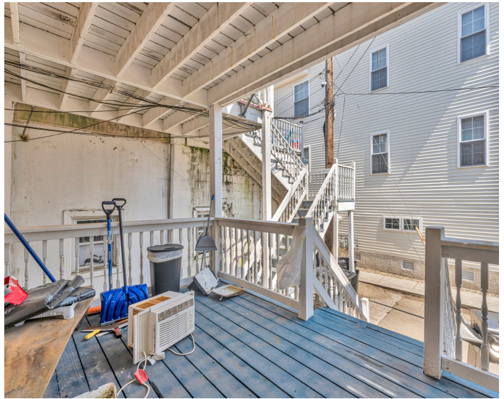
REAR DECK AND ACCESS STAIR
