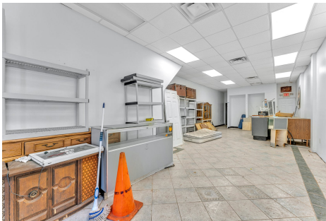
DISPLAY CASEWORK REMAINING
