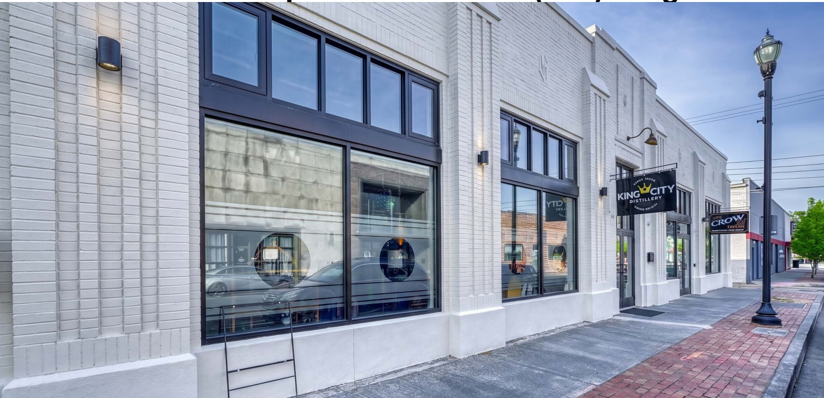
Facade Grant - Potential Renovation
