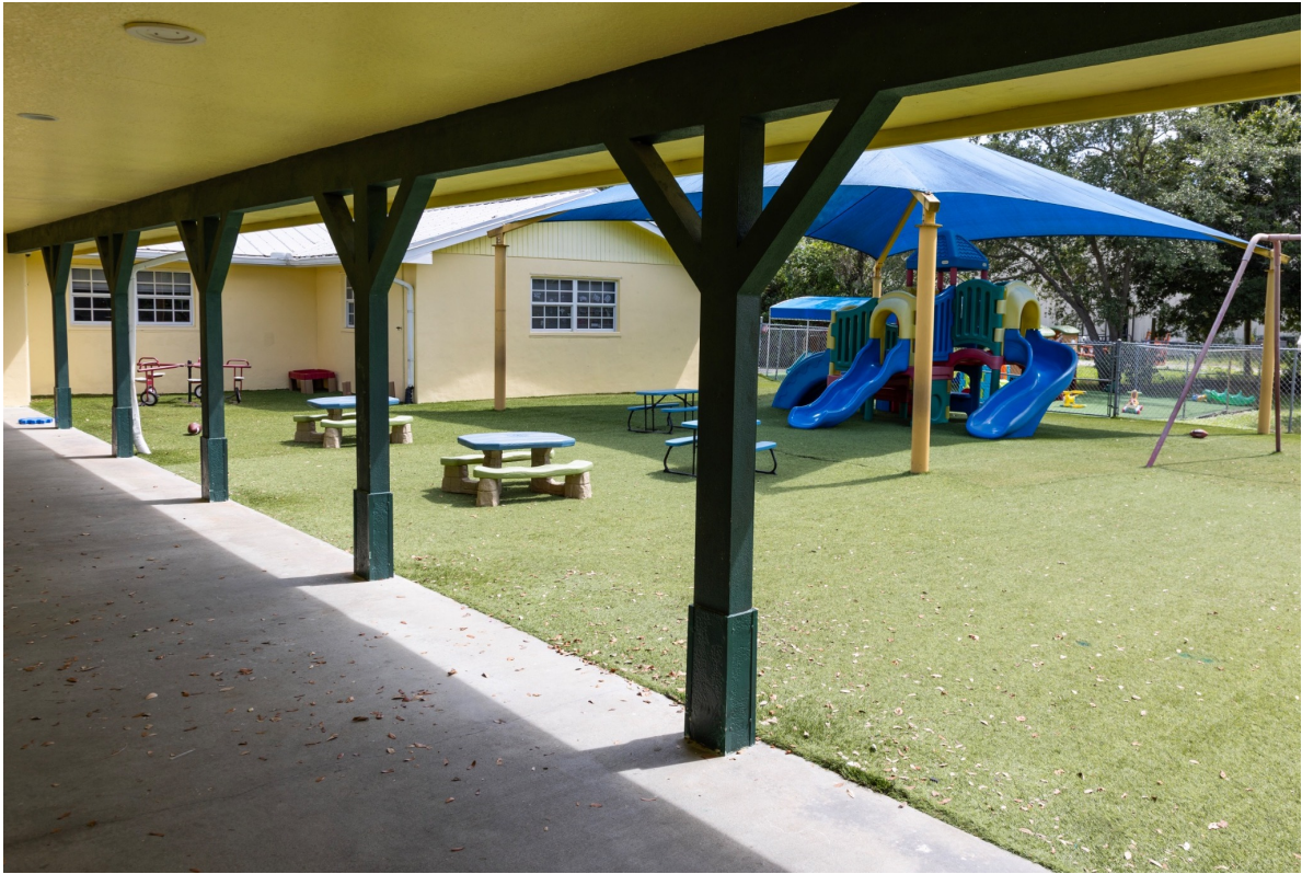
Building, play areas and improvements operate as one childcare campus
