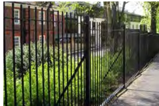
Vertical bar railings to shared garden
