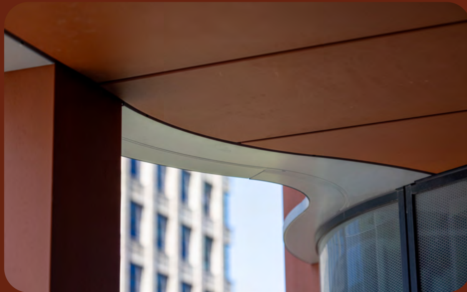
Terrace soffit on Level 3
