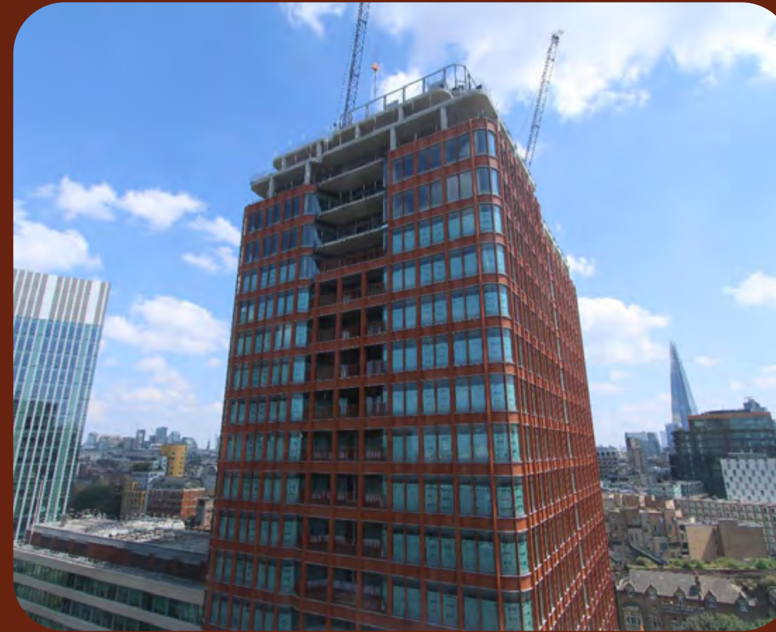
Façade installation up to Level 18
