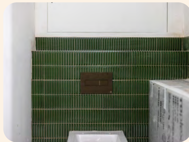
Level 3 super-loo tiling & sanitary-ware
