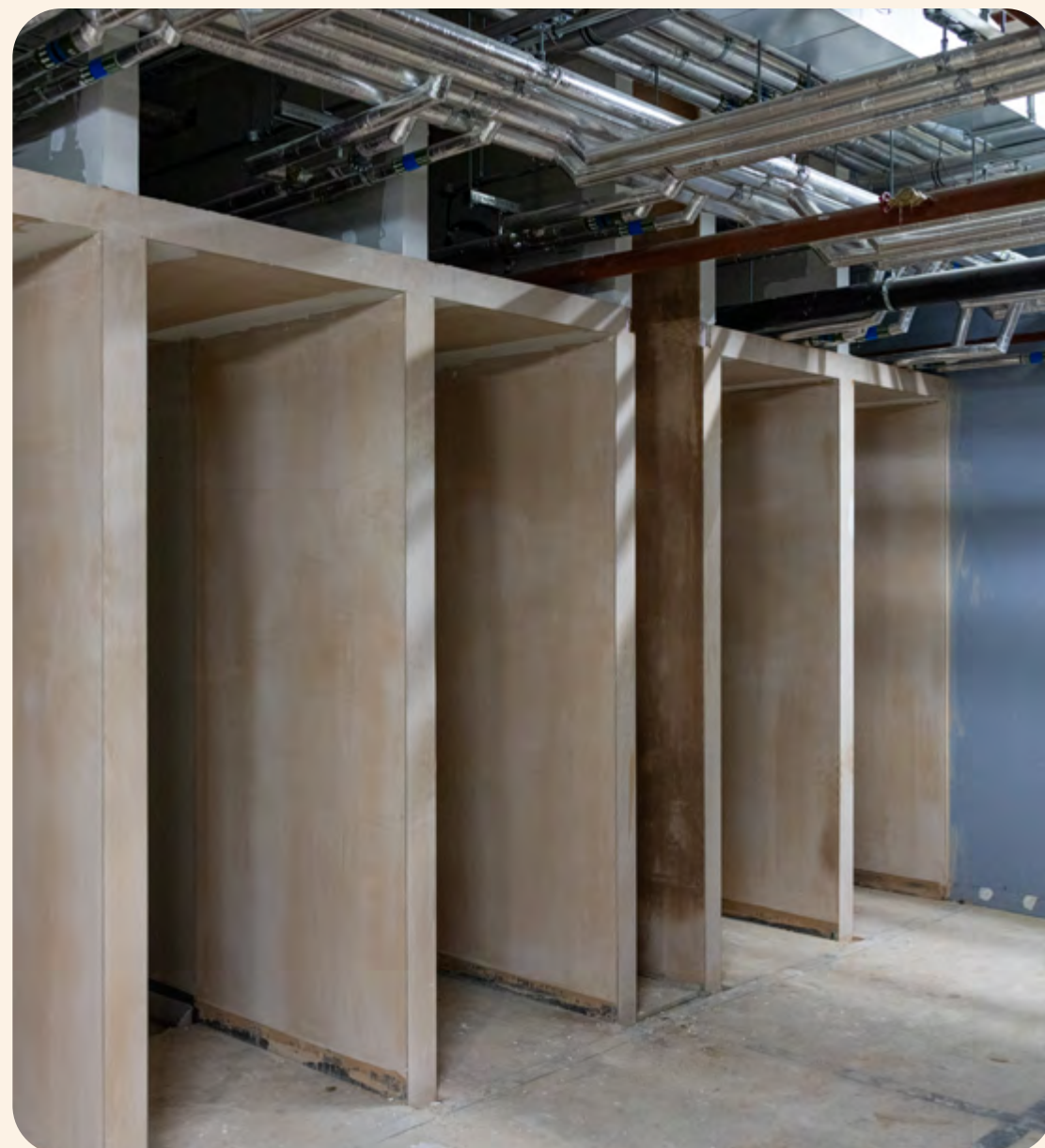
Shower cubicles on Basement -1
