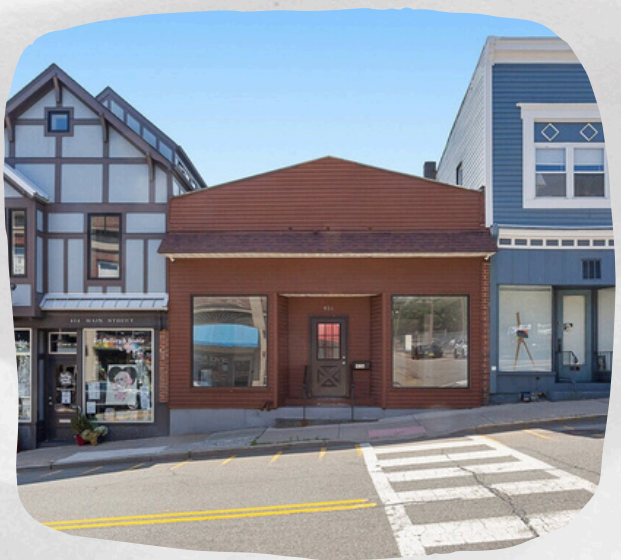
CURRENT CONDITION -FRONT OF 416 MAIN ST
