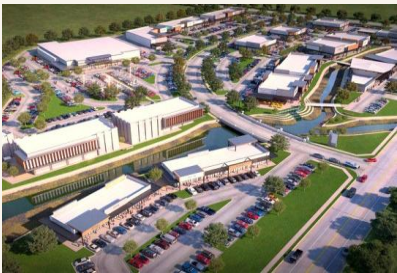
WATER-FRONT CREEK FRONTAGE
