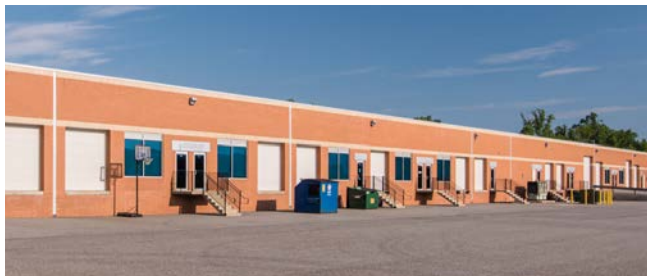
Flex/R&D dock and drive-in loading
