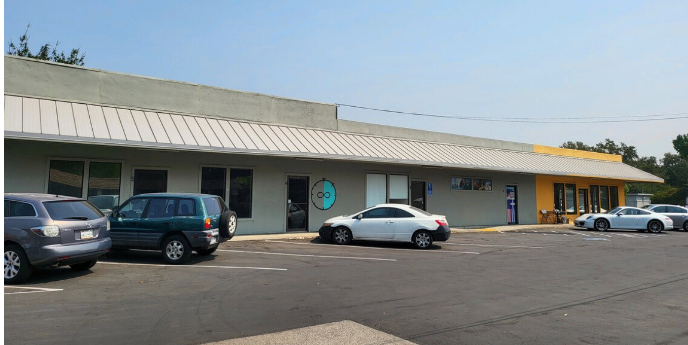
SIDE OF BUILDING
