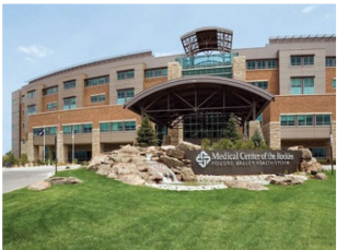
Medical Center of the Rockies Regional Hospital
