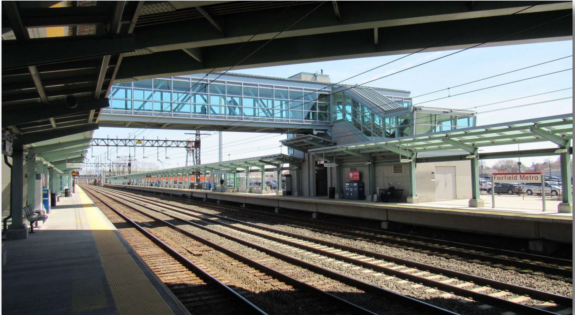
Metro North Train Station Platform Next Door
