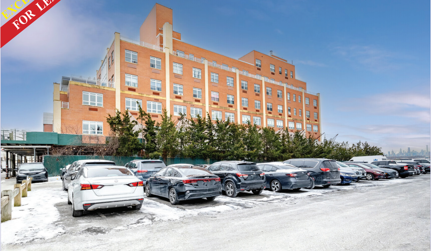
Waterview Plaza is a contemporary 7-story mixed-use building located on the East River/Flushing Bay waterfront in College Point, Queens.
