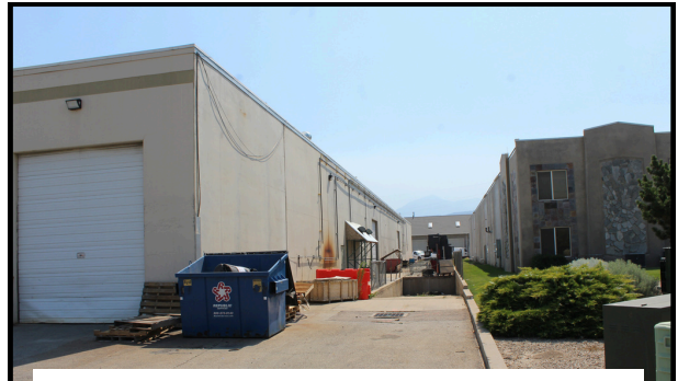
Shared loading dock
