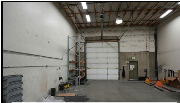
7 ground level doors (12'x14')
