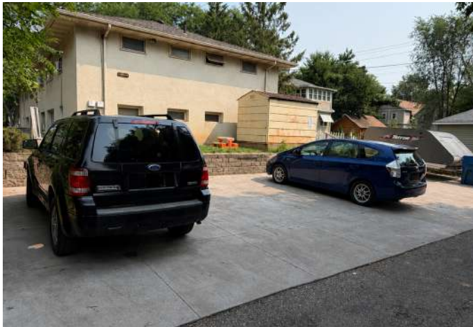
Rear Parking / Common Exterior
