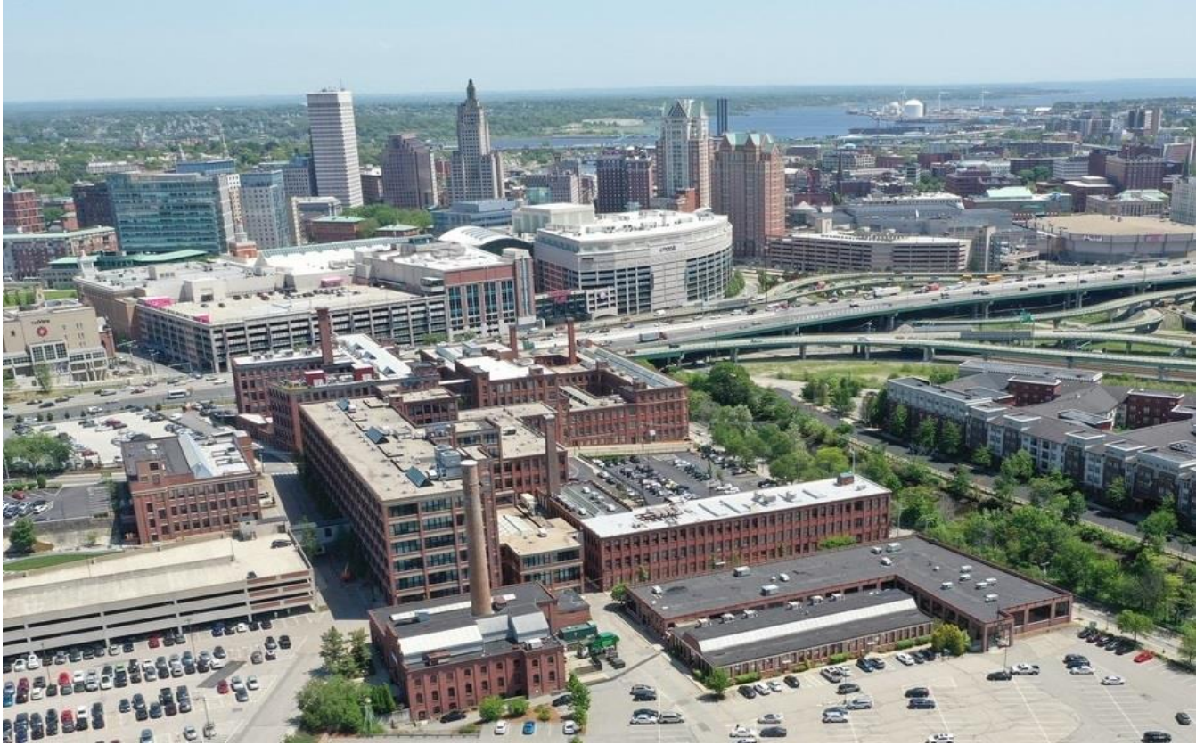
The Foundry aerial view & proximity to downtown Providence, RI.
