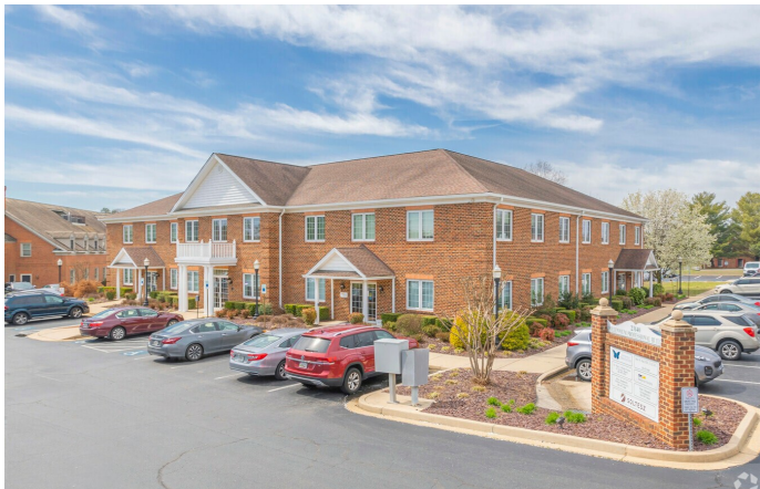
EXTERIOR · EAST ELEVATION
